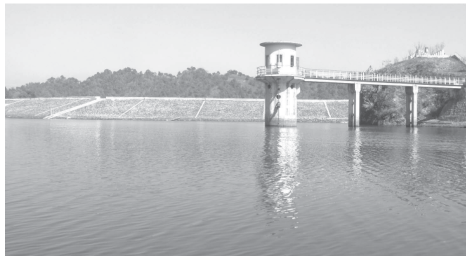
Water control tower of Pyaingchaung Dam.
