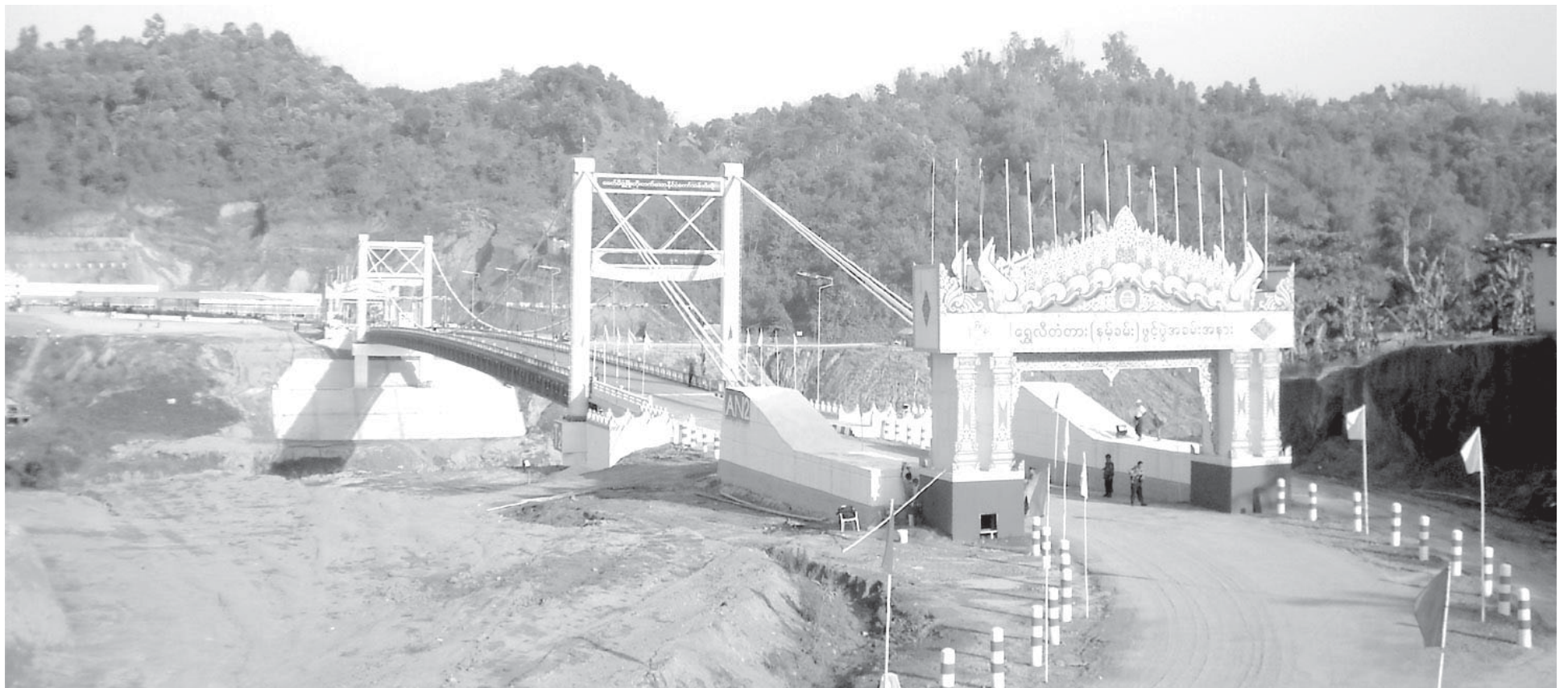
Photo shows Shweli Bridge (Namkham).—CONSTRUCTION
