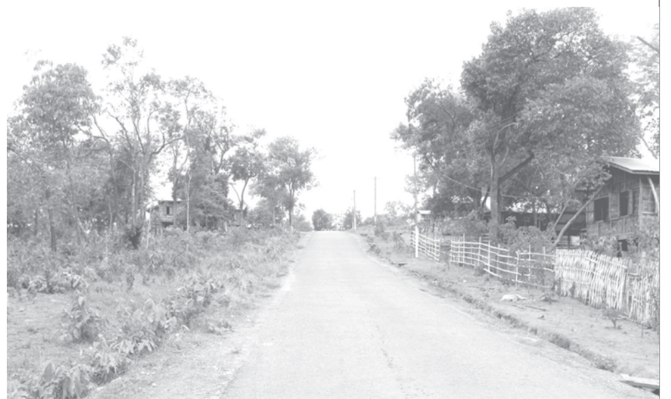
Newly-built streets in Htot-kawkoe village.
