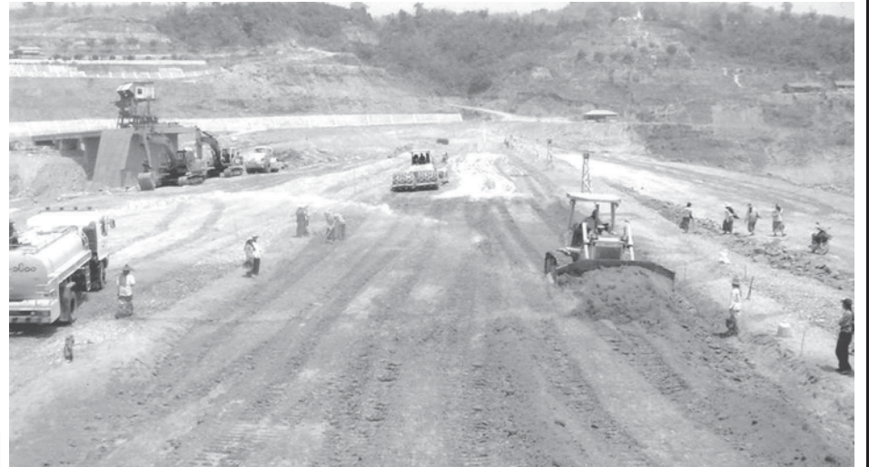
97 per cent completion of main embankment.
