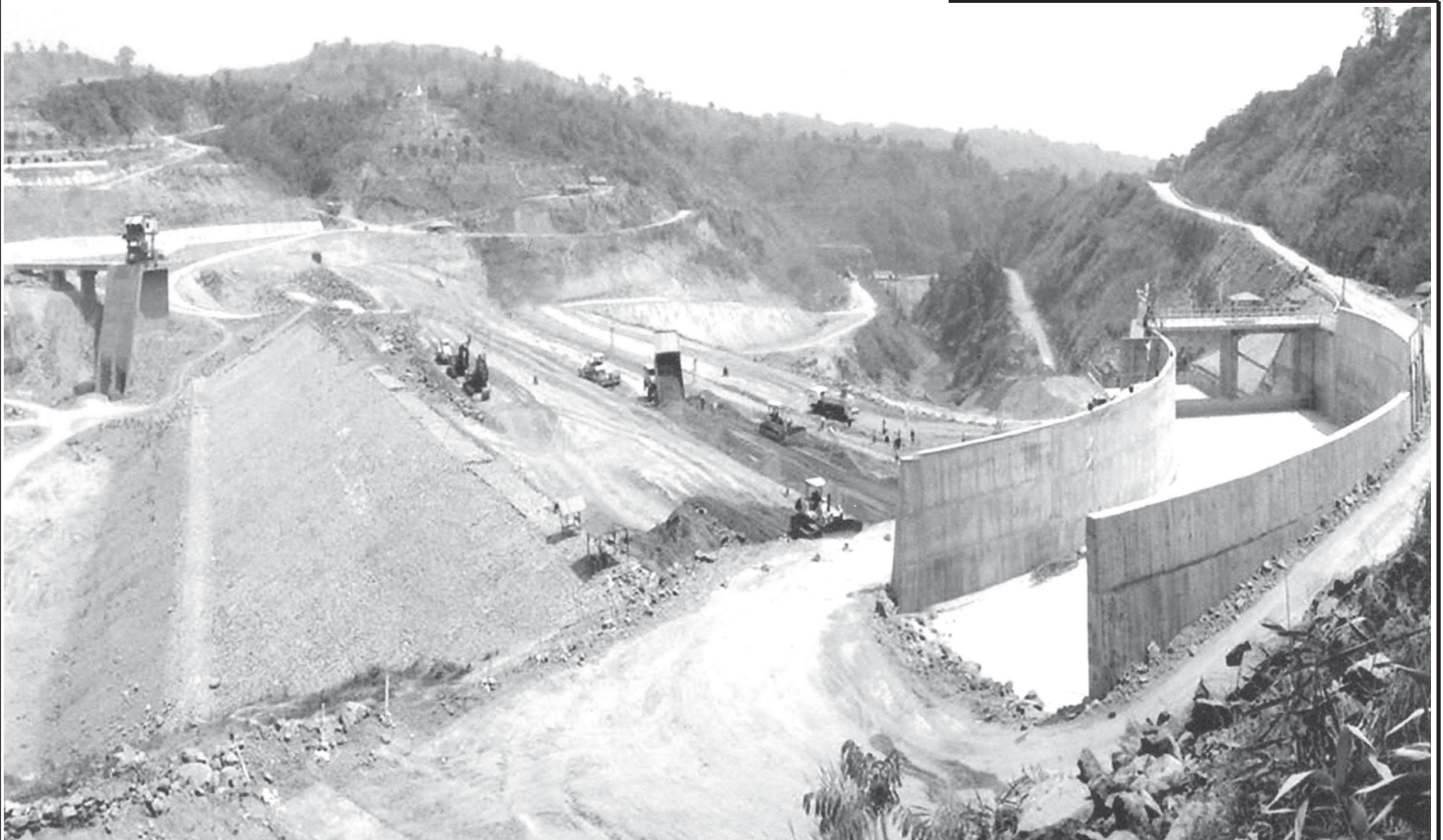
Main embankment and spillway (water intake canal) are under construction in Kunchaung Hydropower Project in Pyu Township of Bago Division.
