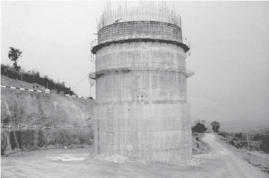
96 per cent completed surge tank at Kunchaung Hydropower Plant.
