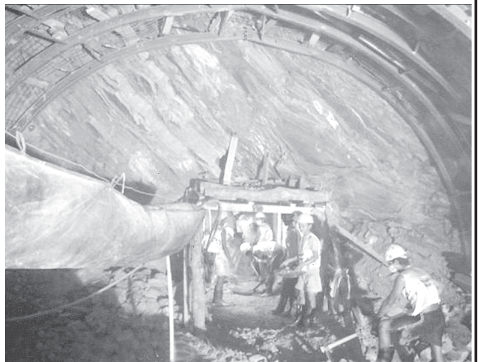
Workers and technicians drilling tunnel exit at Pyuchaung Hydropower Project.
