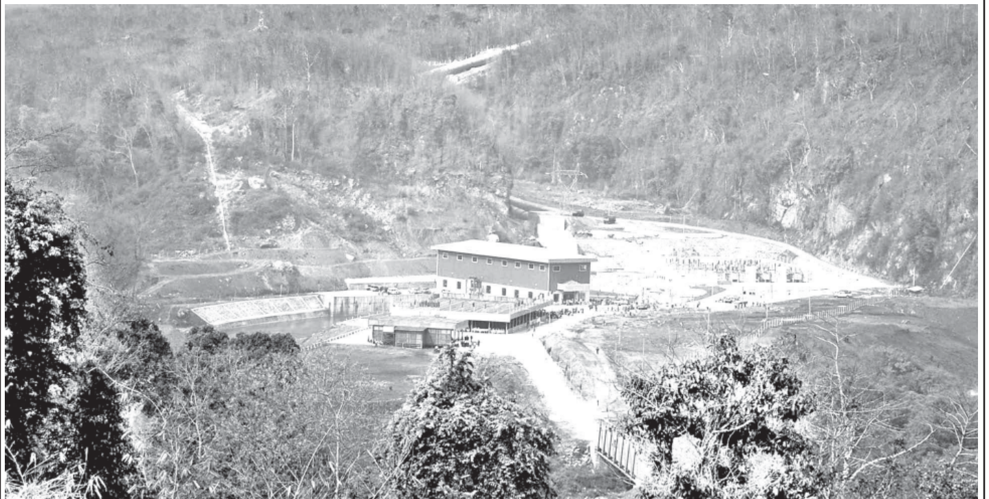
Kengtawng Hydropower Plant in Kengtawng region.
