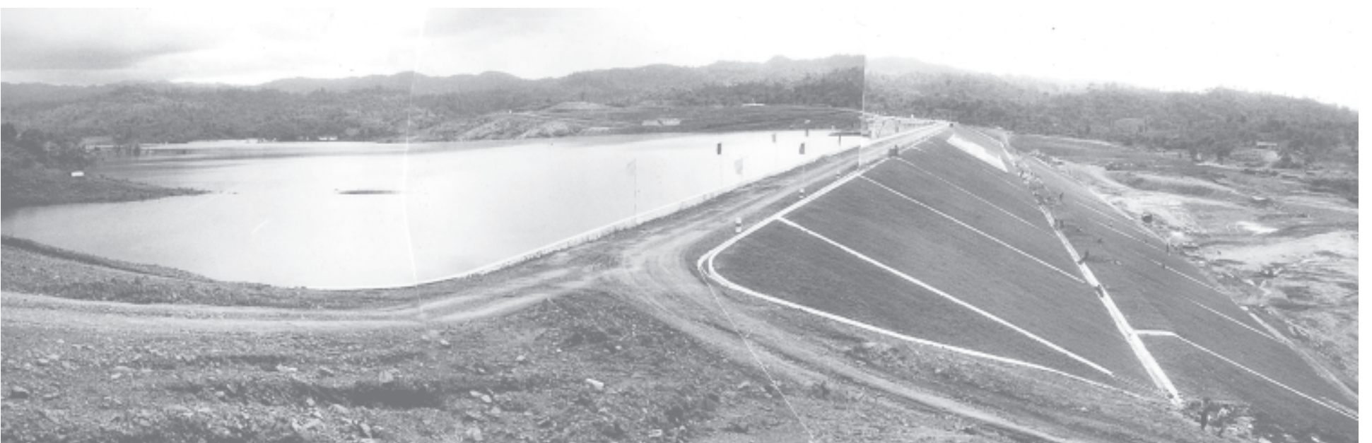
Khawa Dam built by Construction-2 of the Irrigation Department near Chinywagyi, Padaung Township, Bago Division, benefits 2,000 acres of farmland.— MNA
