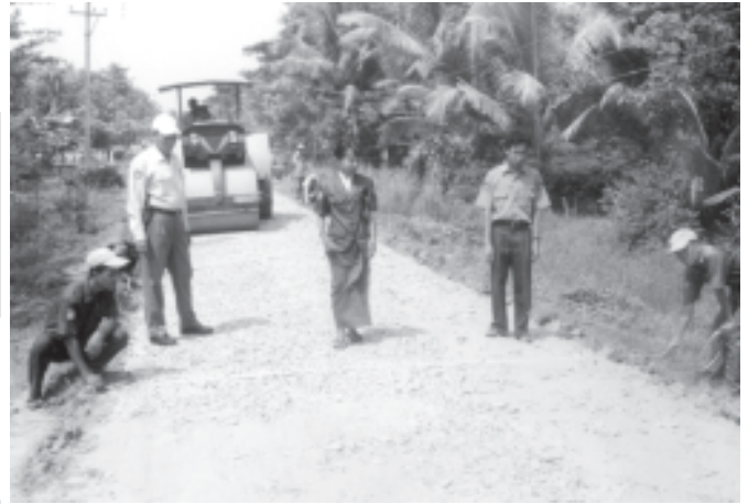
For better transportation in rural areas, roads linking one village and another are being built. The photo shows one of the road construction sites in Nyaungdon Township, Ayeyawady Division.—PBANRDA
