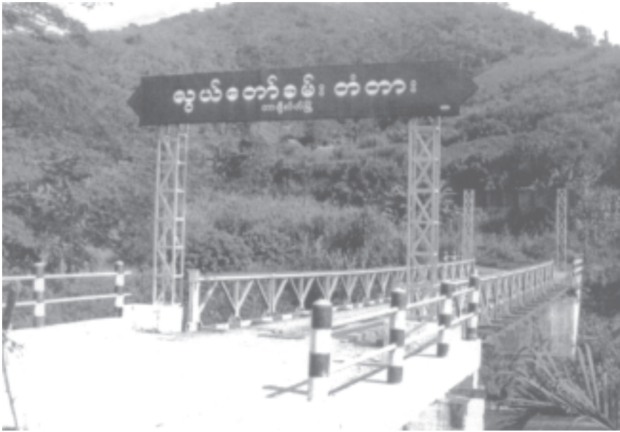
Loitawkhram bridge in Tachilek Township, Shan State (East), contributes much towards the convenience in travelling of local people. — PHOTO: TIN SOE
