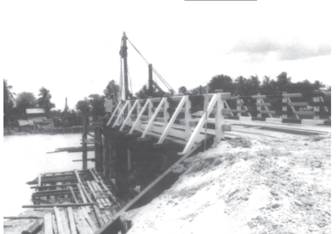
Kyaukchaunggyi bridge which is under construction on Patheingyi road in Ayeyawady Division.— MNA
