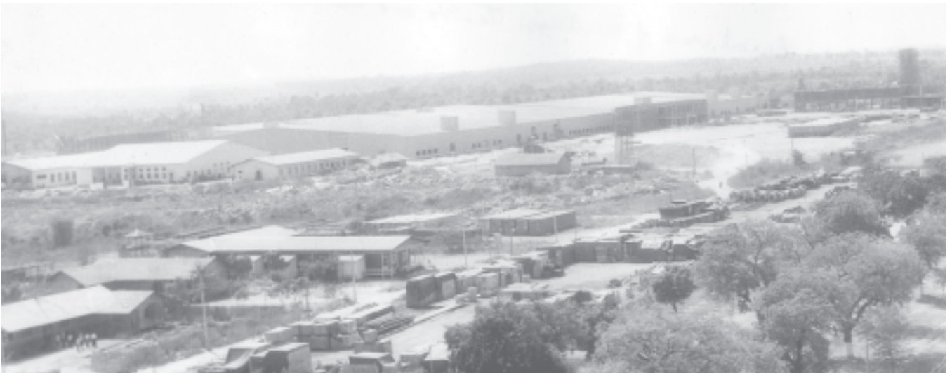
Aerial view of Salingyi Textile Factory Project in Sagaing Division.
