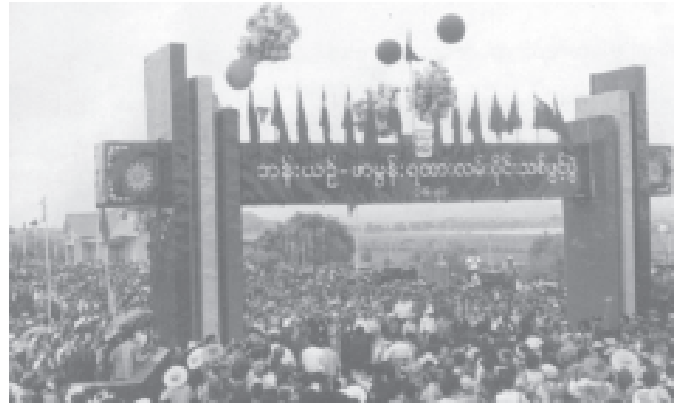
The opening of the Banyin-Phamon Railroad Section in progress in Hsihseng Township, Shan State (South), which was constructed by Tatmadaw members.
