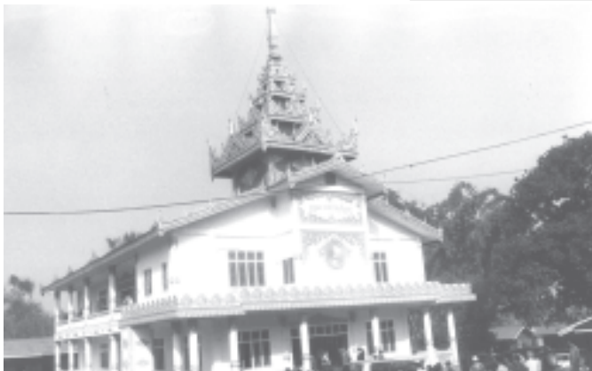
Sasana Jotika Ordination Hall and two-storey refectory of Myole Pariyatti Monastery in Lashio. — MNA
