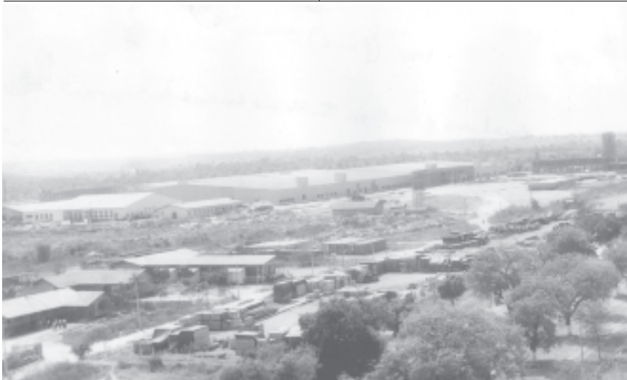
Aerial view of Salingyi Textile Factory Project. (News reported) — MNA
