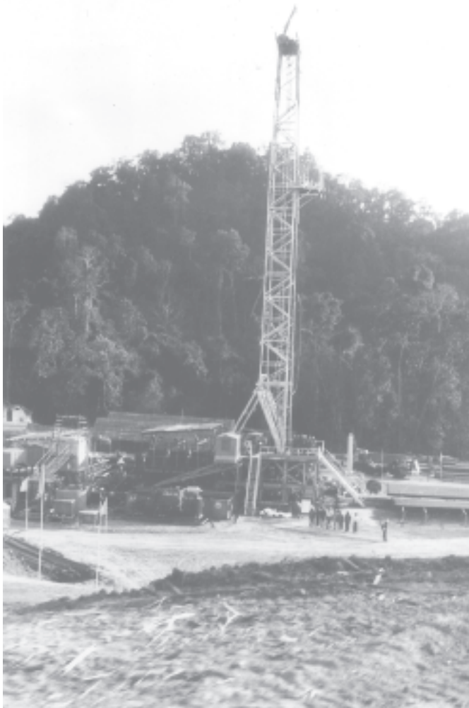
Drilling tasks being carried out at No 3 well in Indaw region, Mawlaik Township.
