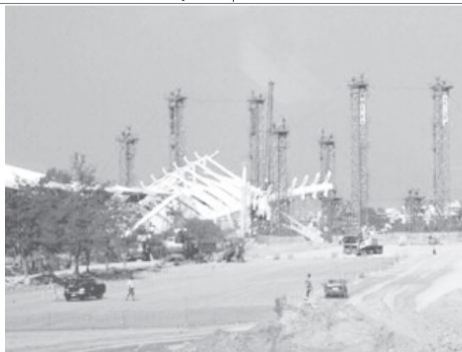
View of the construction site of the velodrome in Athens City which is due to be used in the next Olympics Games 2004 in Athens.
