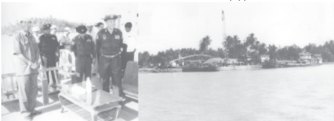
Lt-Gen Khin Maung Than inspects Pyapon Bridge construction project.— MNA
