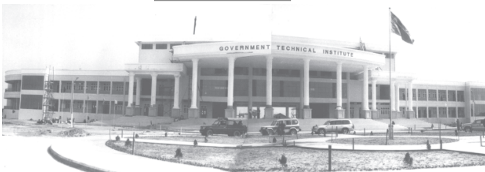
Government Technical Institute (Myingyan) under construction in Myingyan, Mandalay Division seen on 27 January.
