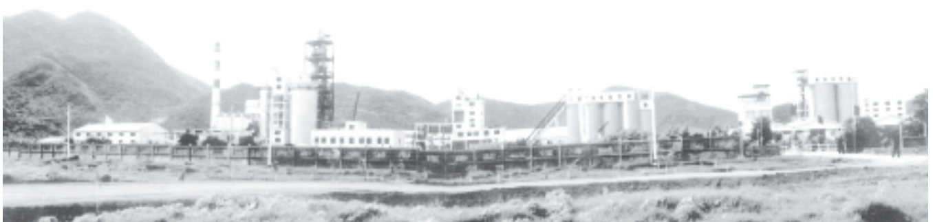
A 500-ton cement plant of the Ministry of Industry-1 in Kyaukse Township.
