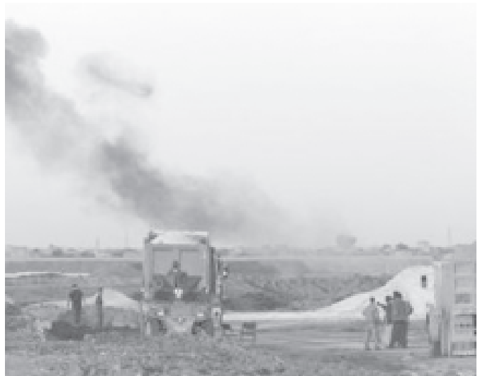
Black smoke rises from the construction site in Samawa, southern Iraq, on 10 Feb, 2004 after the Dutch forces explosive ordnance disposal unit disposed of an explosive.
