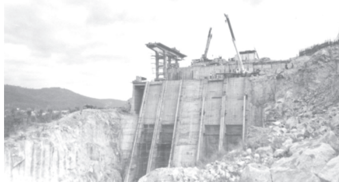
Power Intake under construction at Paunglaung Dam Project.
