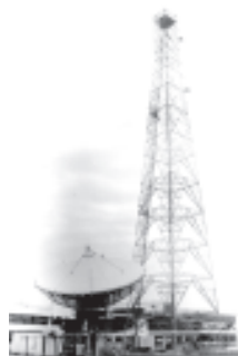
Ground satellite station of Bagan Cybertech in MICT Park.
