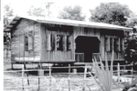
Low-cost rural houses as the one shown in the photo are being built for easing the shelter needs of the village people.
