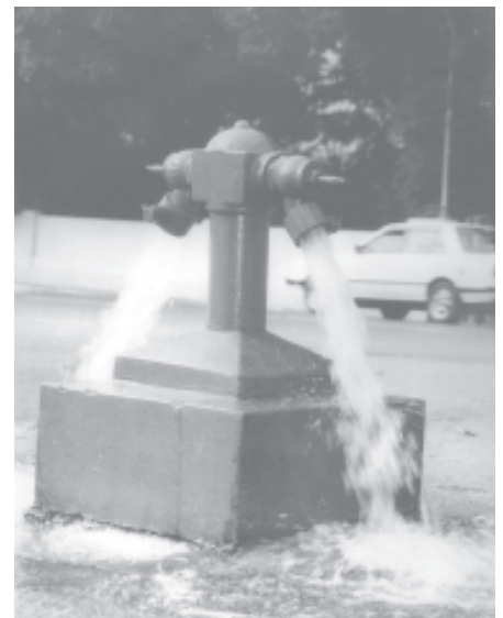
Fire hydrants like the one shown in the picture are ready round the clock to provide water for firefighters in case of emergency need.
