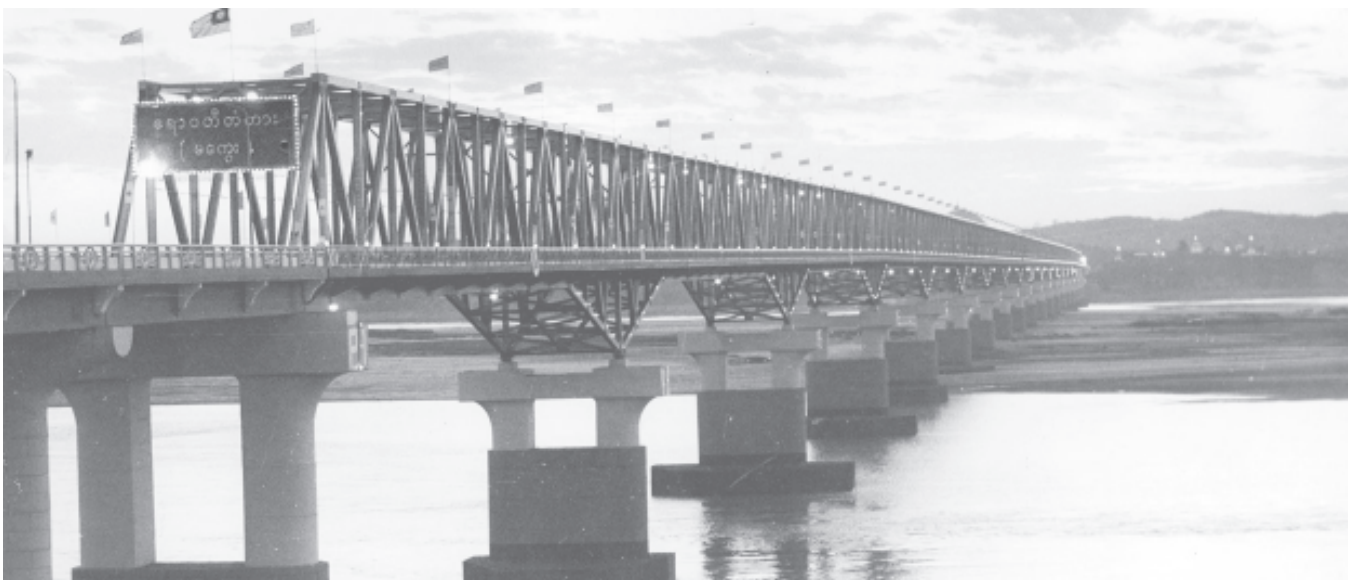
The 8,989 feet long Ayeyawady Bridge (Magway) links Magway and Minbu. The construction of the bridge started on 20 January 2000 and was commissioned into service on 24 November 2002. — PHOTO: MNA
