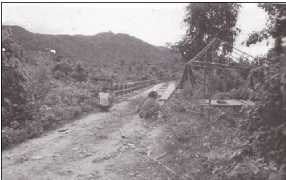
Klaw Maw village, just west of the hills in Kyauk Kyi township, Nyaunglebin District, Karen State. Villagers are taking a break during the forced labor to build a sentry hut, which is half-constructed on the right. [Photo: KHRG researcher]
