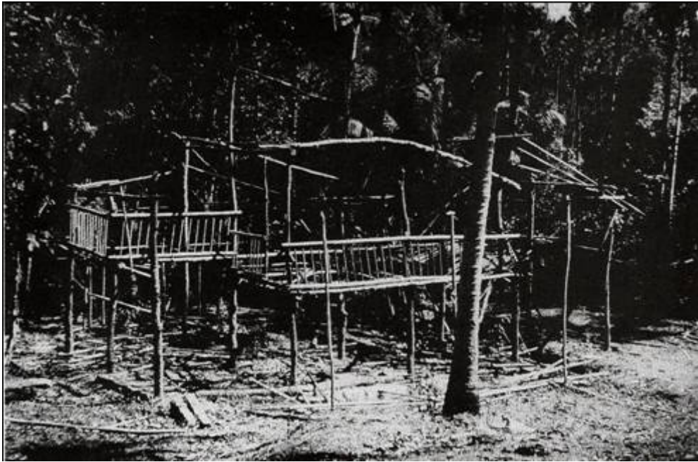
Houses burned and destroyed in Wah Thu Lo village as SLORC tried to force the villagers to move to Ka Pyaw relocation site. (Photo by KHRG)
