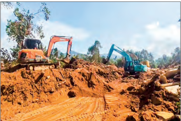
Heavy machinery in use to remove and clean the landslide area in Taninthayi Region.
