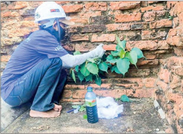
A Future Bagan member injects chemicals to remove plants growing on an ancient pagoda in Bagan.
