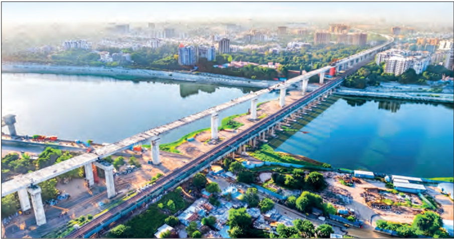
The newly completed Sabarmati River bridge stands approximately 36 metres tall.
