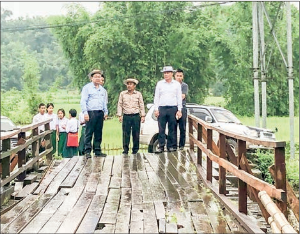
Officials inspect the construction site of a reinforced concrete bridge near Makyawtwah Village, PutaO Township, yesterday.
