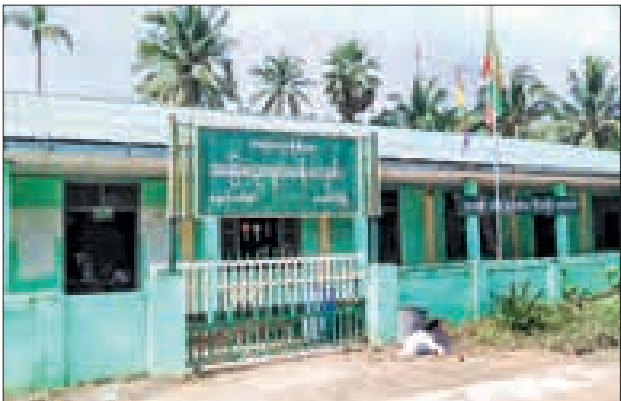
This photo features a school in Taninthayi Region that was temporarily closed due to flooding and has since reopened.
