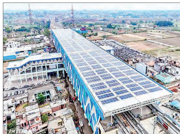
The image shows an aerial view of the Meerut South RRTS station on the Delhi-Meerut Regional Rapid Transit System (RRTS) corridor, featuring a large rooftop solar power plant.
