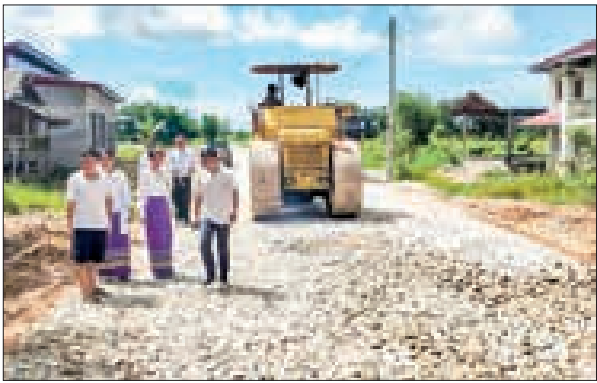
Officials oversee the concrete pavement work in Myeik Township, Taninthayi Region. is being implemented by Htoo Htoo Htet Co Ltd and commenced on 20 August. The project has so far been 50 per cent complete. Upon completion, the road is expected to enable agricultural produce from 1,848 acres of farmland in Kywegu Village to be transported to markets more quickly, according to the Myeik District Department of Rural Development. — Ah Htwe (DRD)
