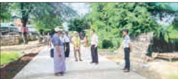
Officials inspect the concrete paving work in Minbu Township, Magway Region.
