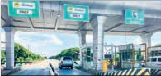
A toll gate on the Yangon-Mandalay Expressway with the TollPass RFID system.
