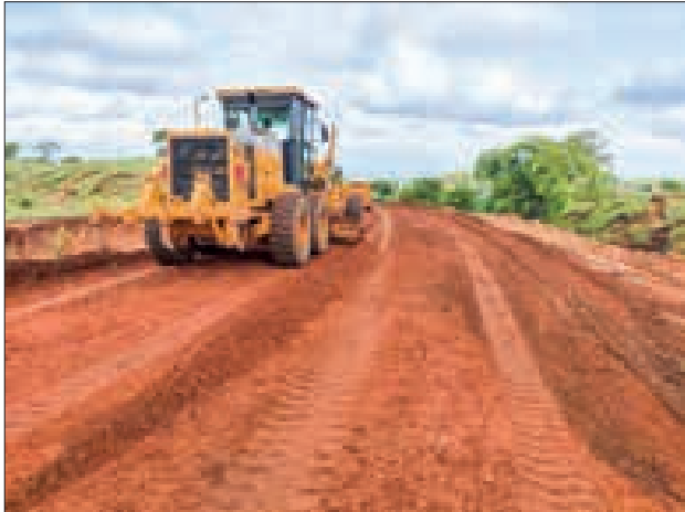
This image captures the laterite paving work in Yenangyoung Township.
