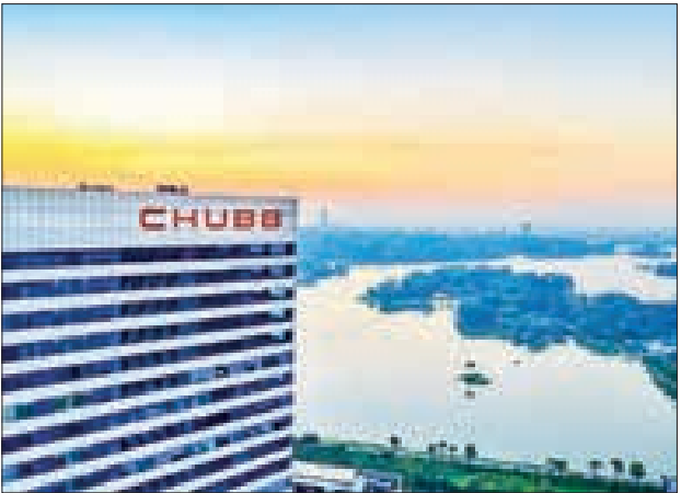
A general view of the CHUBB Life Myanmar Insurance Company building. the state-owned Myanmar Insurance also provides insurance services. — ASH/MKKS
