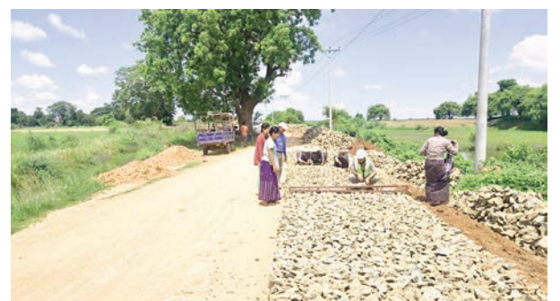
Officials inspect the concrete paving work on the Chinhtaung-Kyauksan Road in Minbu Township.
