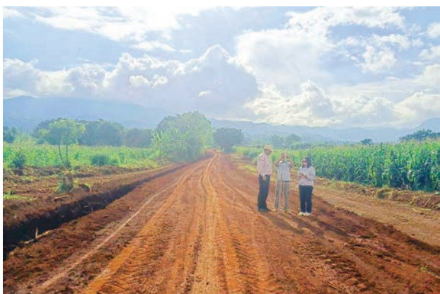
A field inspection is underway in Taunggyi Township, southern Shan State.
