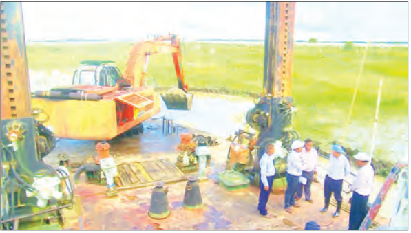
Machinery being operated in repairing Toe River embankment in Nyaungdon Township.
