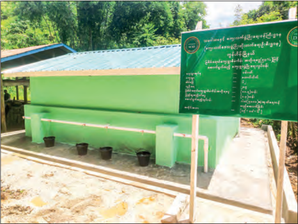
This image shows the completed water tank project in Kunhing Township.
