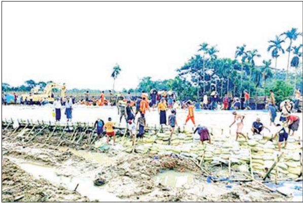
Riverbank protection measures taken in Nyaungdon Township.
