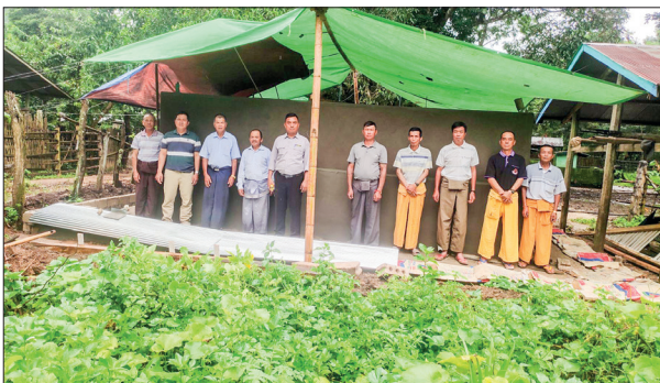
Officials and residents are seen during the inspection of the 5,000-gallon water tank construction in Kunhing Township.
