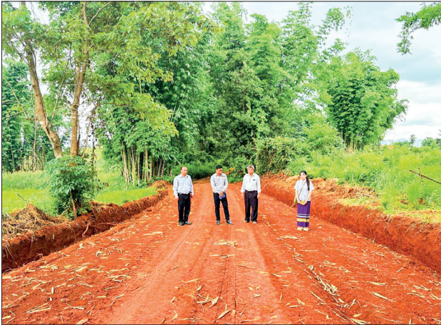
Officials oversee the construction progress of a rural farm-to-market road in Mongnai Township.
