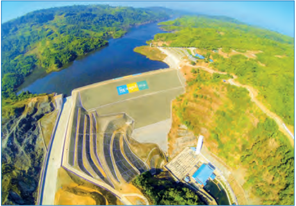
An aerial drone view of the Pyu Creek Dam and its surrounding areas. further: Pyu Creek Dam generates electricity throughout hot, rainy and cold seasons. Depending on water inflow, when water availability is sufficient, the plant can generate up to 800 megawatt-hours, making the dam beneficial to the country,” said U Min Thu Aung, Manager of the Pyuchaung power plant. The Pyuchaung Hydropower Plant measures 130 feet in length, 110 feet in width and 110 feet in height. Its turbines are Francis vertical-shaft type turbines, with a discharge rate of 2,031.65 cubic feet per second. The plant has two 20-megawatt generating units and produces an annual average of 120 million kilowatt-hours of electricity, which is transmitted to the national grid through the 230-kV Toungoo power line. The dam stores and regulates water flowing from the Bago Yoma and also supports the agriculture and livestock sectors in Pyu and Ottwin townships. It helps prevent flooding in the Sittoung River basin and provides water needed by farmers in Pyu and Zeyawady for summer cultivation. Construction of the Pyuchaung Hydropower Plant began in 2001 and was completed in August 2014. Since 29 August 2014, the plant has been supplying electricity to the national power grid through its two 20-megawatt generating units. The dam is not only a major facility for electricity generation but also an important reservoir supporting the agricultural sector. — Thitsa (MNA)/KTZH
