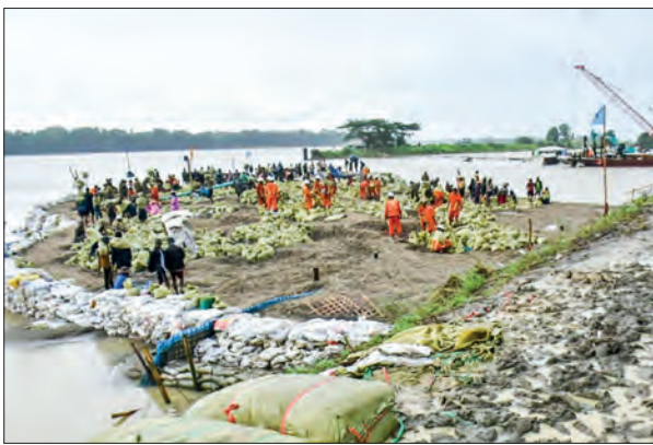
Officials inspect preparation to block water inflow in Laymyethna Township.
