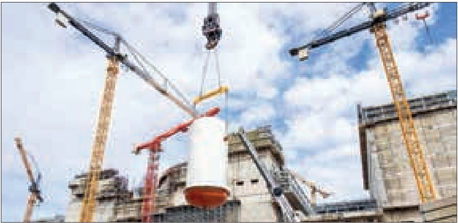
Heavy crane installs key reactor component at Akkuyu Nuclear Power Plant in Türkiye, constructed by Russia's Rosatom. PHOTO: ATOMIC ENERGY 2.0
