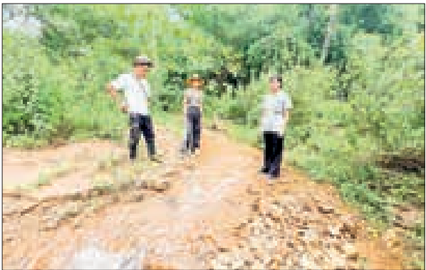
Officials inspect an ongoing spring water supply project in Kehsi Township in southern Shan State. source to Nayok Village. She also met representatives of the tender-winning company, urging them to complete the project on
