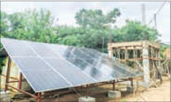
This image displays the construction site of the elevated water tank.
