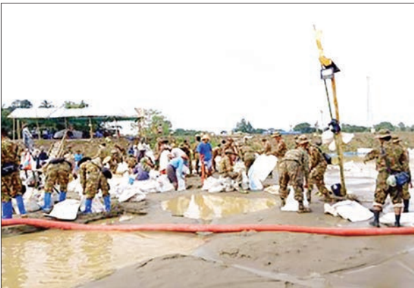
This image shows ongoing floodway closure works in Laymyethna Township.
