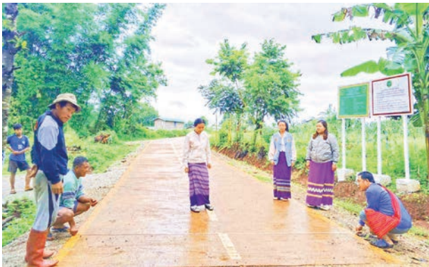
Officials oversee the completed road construction project in Hopong Township.
