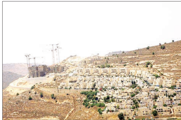
This photo taken on 9 August 2026 shows an Israeli settlement under construction in the West Bank, near Jerusalem. PHOTO: XINHUA
