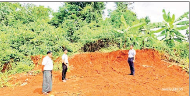
Officials inspect the implementation of a spring water supply project in Mongyang Township.
