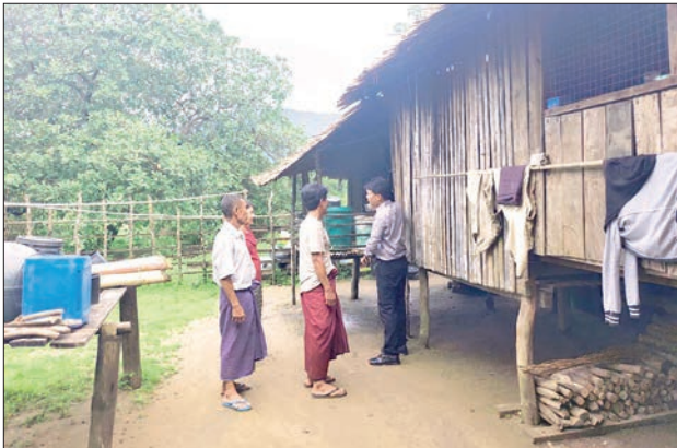
Officials oversee a spring water pipeline installation project in Yebyu Township, Taninthayi Region.
