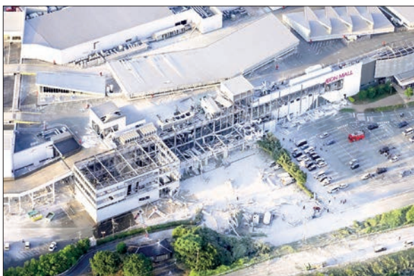
This photo from a Kyodo News helicopter shows an Aeon Mall complex in Kashima, Kumamoto Prefecture, that was extensively damaged following a powerful earthquake that struck the region on 28 July 2026. PHOTO: KYODO
