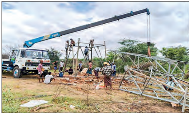
Repair works underway on the collapsed 132kV Nyaungbingyi-Buddhagon Tower 338, destroyed in a terrorist bomb blast.
