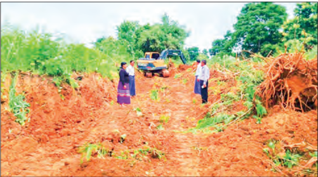
Officials inspect the road construction progress in Sinbaungwe Township.
