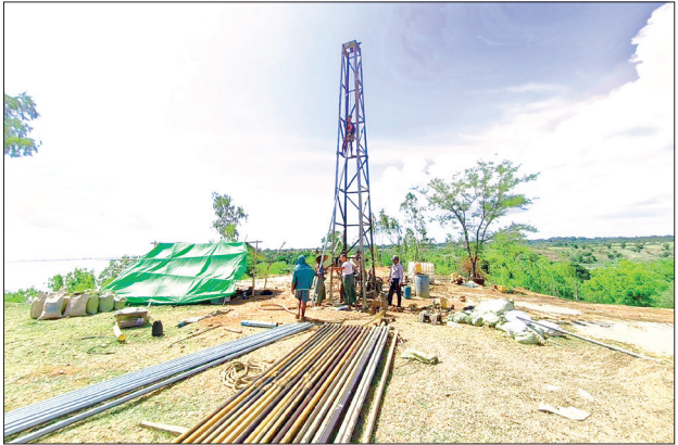
This photo shows a well-drilling rig at the solar-powered water supply project in Yenangyoung Township.
