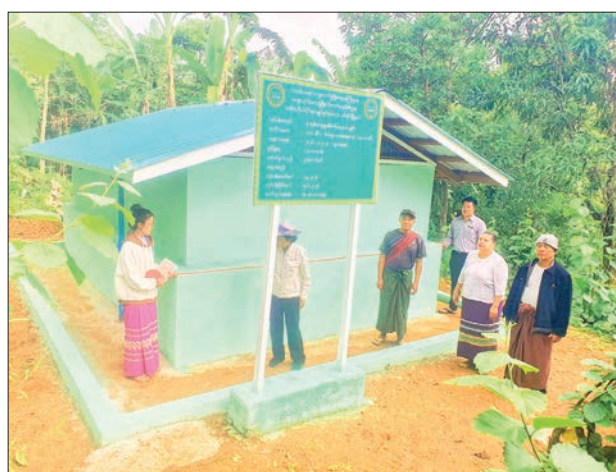
Officials oversee the completed spring water supply system and water storage tank in Hsihseng Township.
