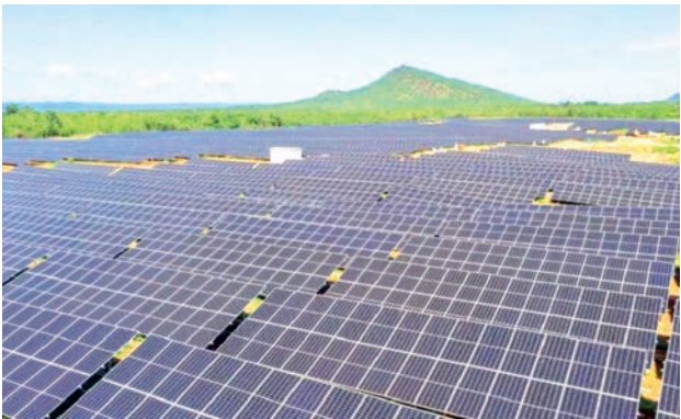
A solar project underway in Myanmar.
