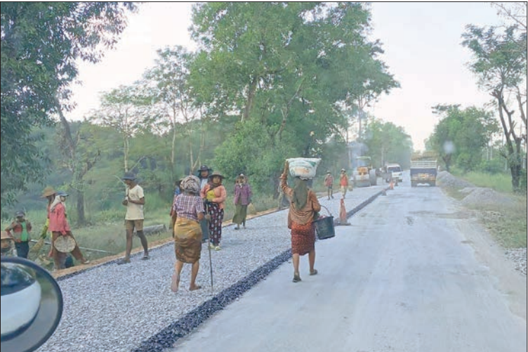
Road upgrading work underway on the Yangon-Pathein Highway between Kankalay and Dahka.
