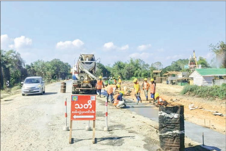
Concrete widening work along the asphalt shoulder at Milepost 59 on the Yangon-Pathein Highway.
