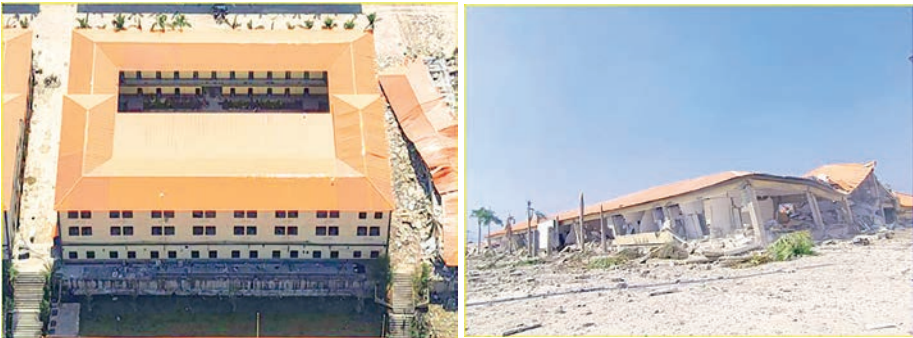
Images show the illegally built three-storey flats before and after the demolition.
