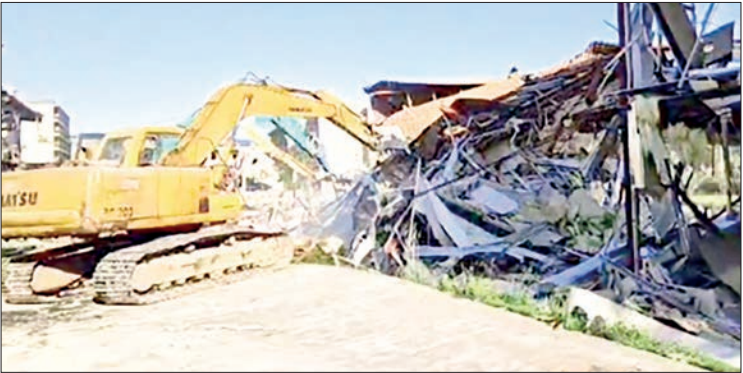
This image captures the demolition measures ongoing in the KK Park Section 3.
