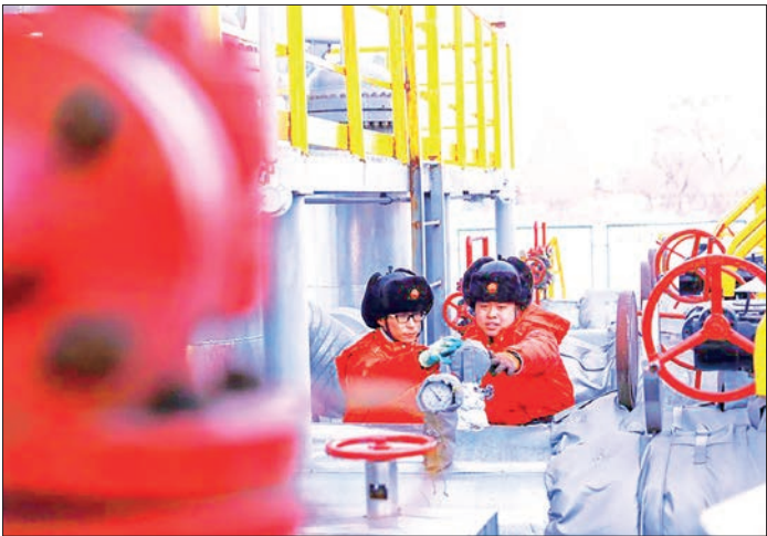
Workers conduct an airtight check at a natural gas company of Daqing Oilfield in northeast China’s Heilongjiang Province, 3 January 2025. PHOTO: MA KE/XINHUA
