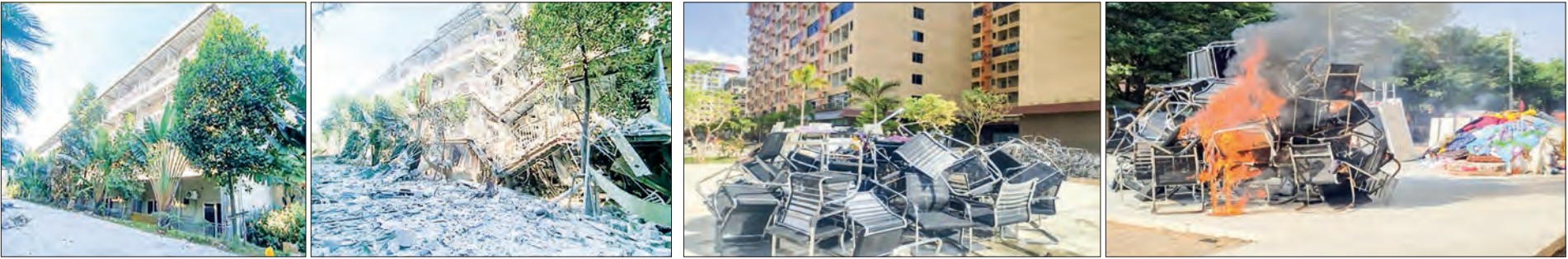
(From Left to Right), The images show demolished building in KK Park Section 3, as part of ongoing demolition measures and the burning of materials used by undocumented foreign entrants in Shwe Kokko, Myawady, Kayin State.
