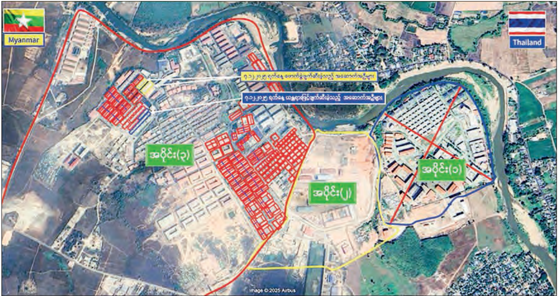
This image reveal the demolition measures underway in the KK Park Section 3, Myawady, Kayin State.
