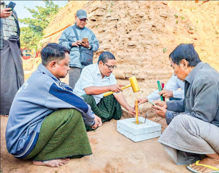
This image displays the foundation plaques being laid for the Inwa tooth-relic building reconstruction.
