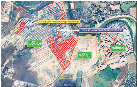
The demolition measure taken at KK Park area 3.
