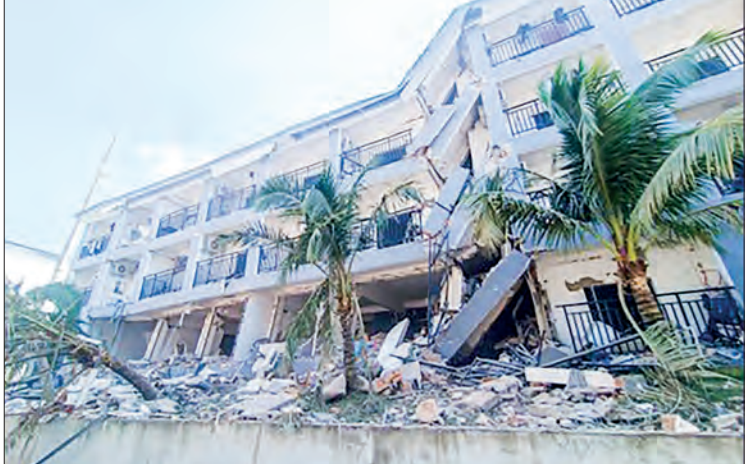
Images reveal the ongoing demolition of illegal housing facilities.
