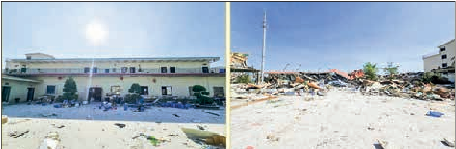
Images show the two-storey facility before and after the demolition in the KK Park area.
