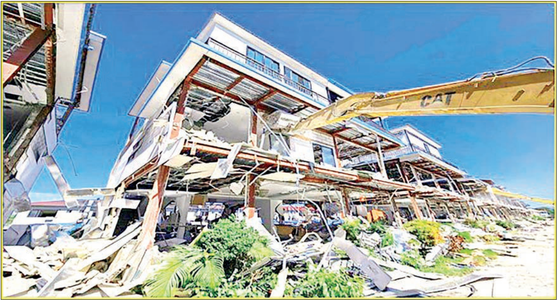
This image shows the demolition of a three-storey building in the KK Park area.
